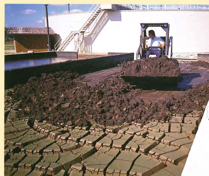
Sludge removal by Front-end Loader
