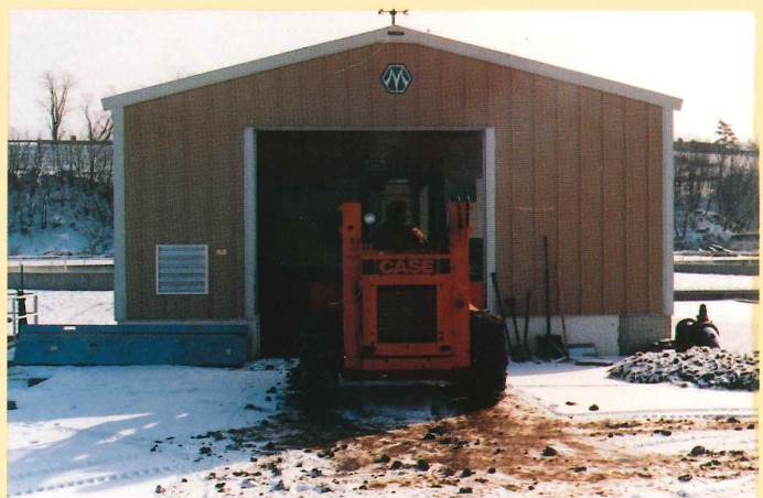
Typical Bed Enclosure over a VSDB at Geneva, Illinois.
